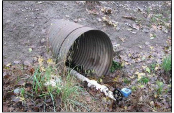
Pipes Through the Levee:
