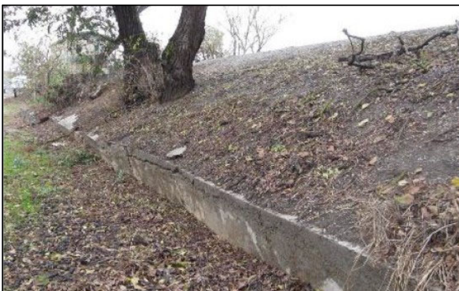
Encroachments Near the Levee:
