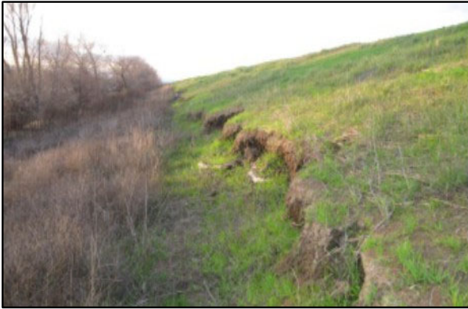
Erosion of Levee Slopes:
